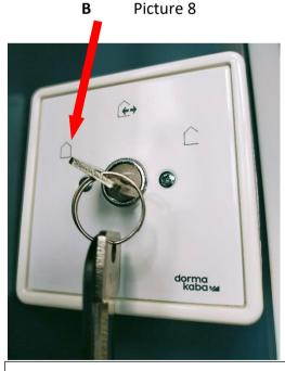
Locked: can <u>only</u> be opened from the inside by pushing the green exit button.
